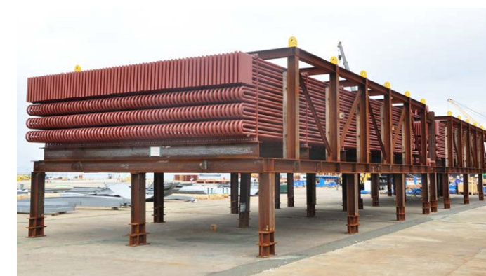
Module assembly of an Economizer for the Mong Duong II Project
