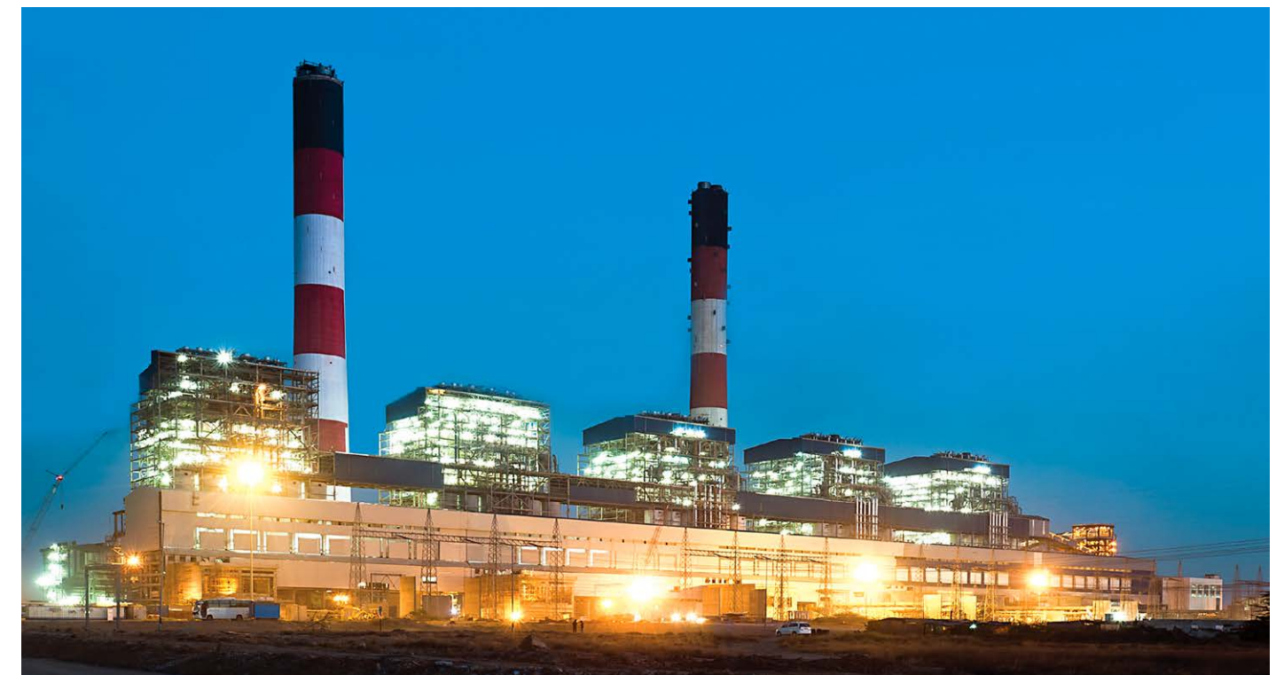
Tata Power's Mundra UMPP is a coal-fired thermal power project with a combined power output of 4,000 MW by Doosan
