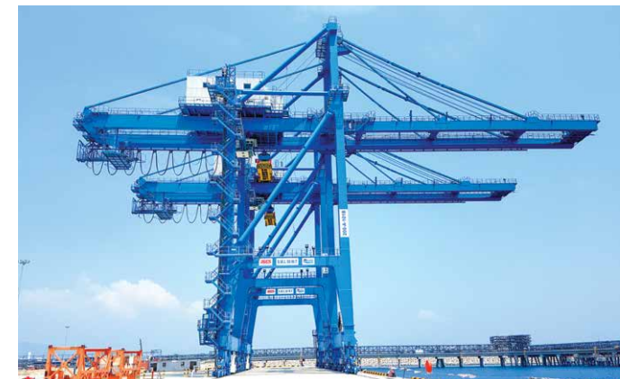
Panamax Cranes at the site of NSRP (Nghi Son Refinery & Petrochemical complex), Vietnam
