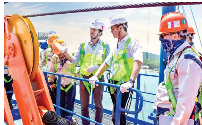
Customer is checking after erection
