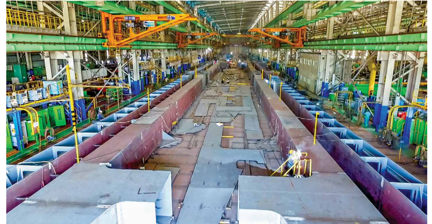
The legs of an RMQC being manufactured in the indoor fabrication area
