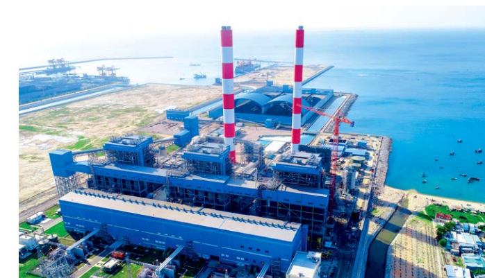
Construction at Vinh Tan IV Power Plant, Vietnam
