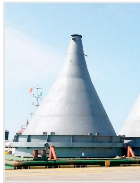
A Coal Silo
