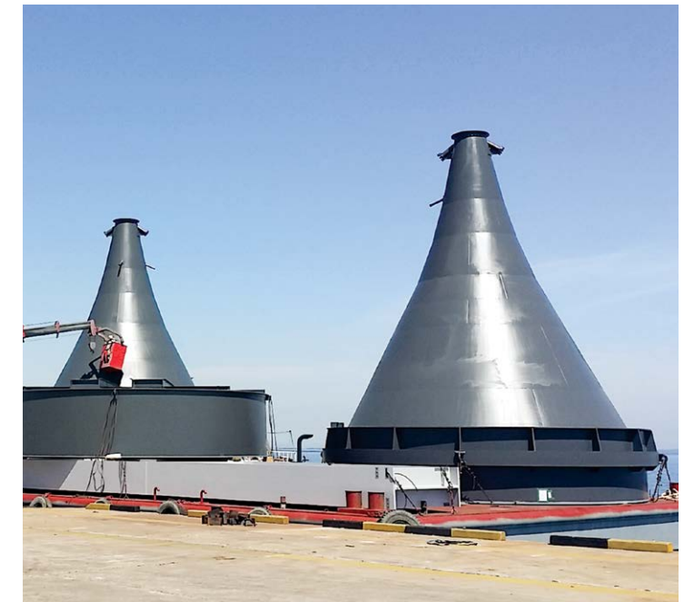
Outdoor assembly of coal silo
