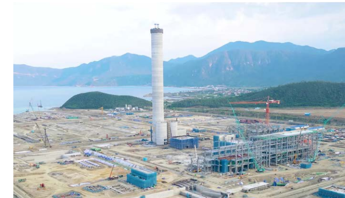
Erecting Steel Structures at the Van Phong Power Plant Site, Vietnam
