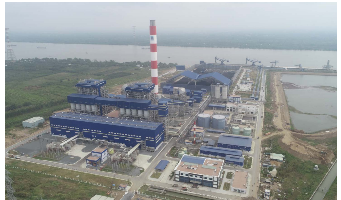
Song Hau I, a 1,200 MW Power Plant in Hau Giang Province, Vietnam completely built by Doosan Vina
