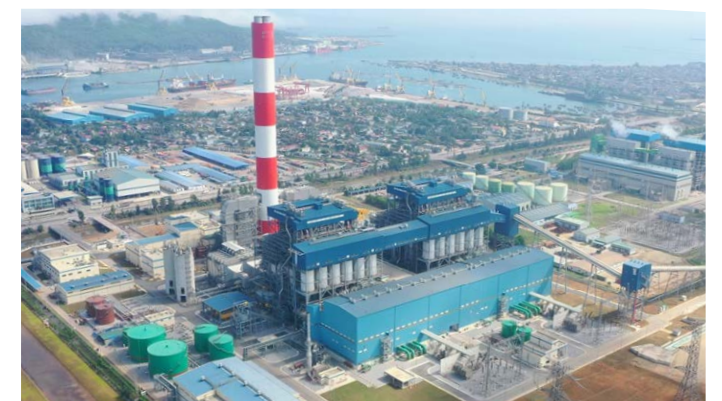
Construction at Nghi Son 2 Power Plant, Vietnam
