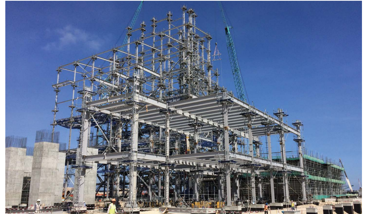
Structural steel products at Vinh Tan IV Power Plant Site, Vietnam
