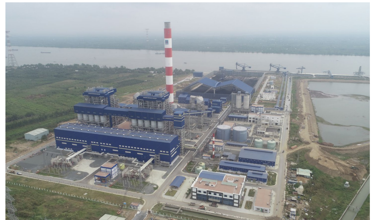
Song Hau I, a 1,200 MW Power Plant in Hau Giang Province, Vietnam completely built by Doosan Vina
