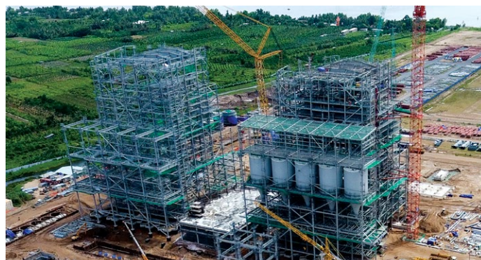
Erecting Steel Structures at the Song Hau I Power Plant Site, Vietnam
