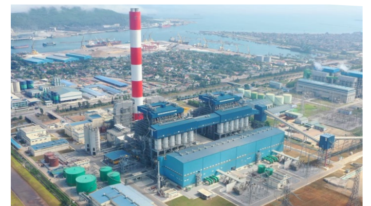
Construction at Nghi Son 2 Power Plant, Vietnam
