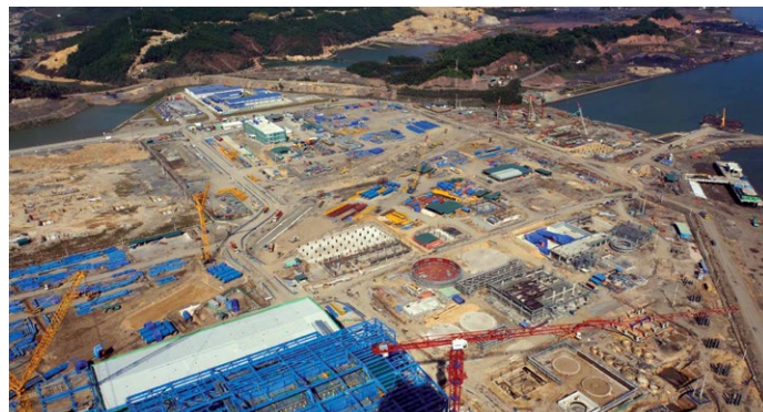
Erecting Steel Structures at the Mong Duong II Power Plant Site, Vietnam
