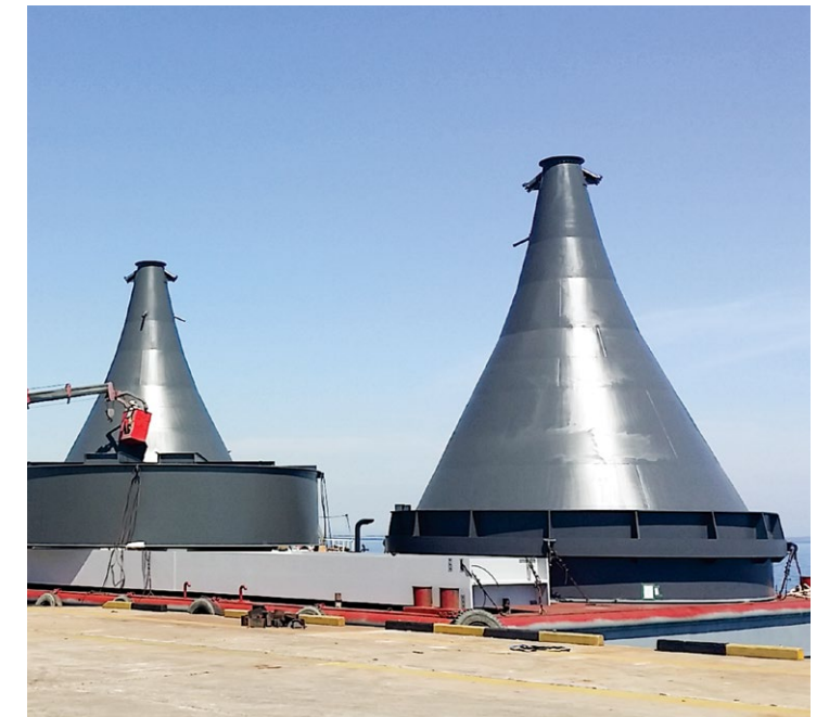
Outdoor assembly of coal silo
