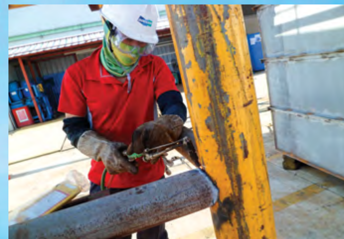
Welding to assemble the new fuel depot
