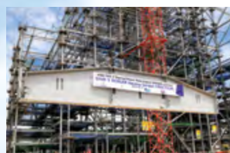
VT4 Boiler support beams are lifted
