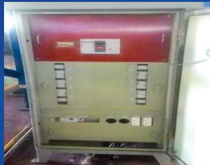
MD15 welding cabinet before and after the first place Keson to upgrade from 400A to 1000A
