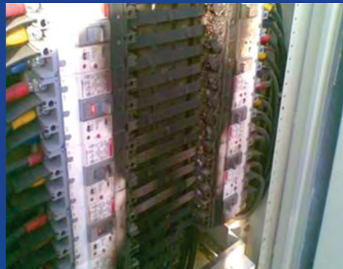
MD15 welding cabinet before and after the first place Keson to upgrade from 400A to 1000A
